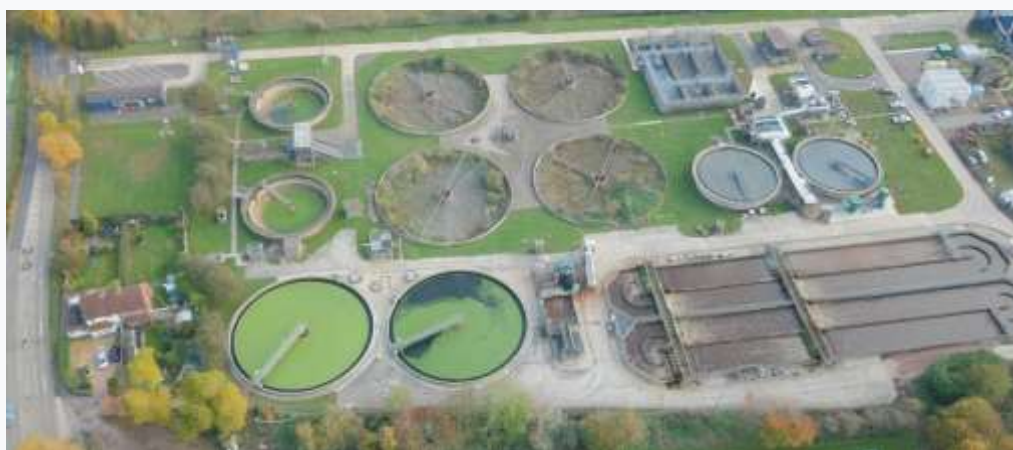
A sewage treatment plant (UK)
