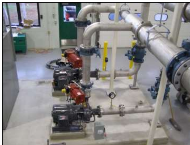
Turbine installation in UK water treatment works
