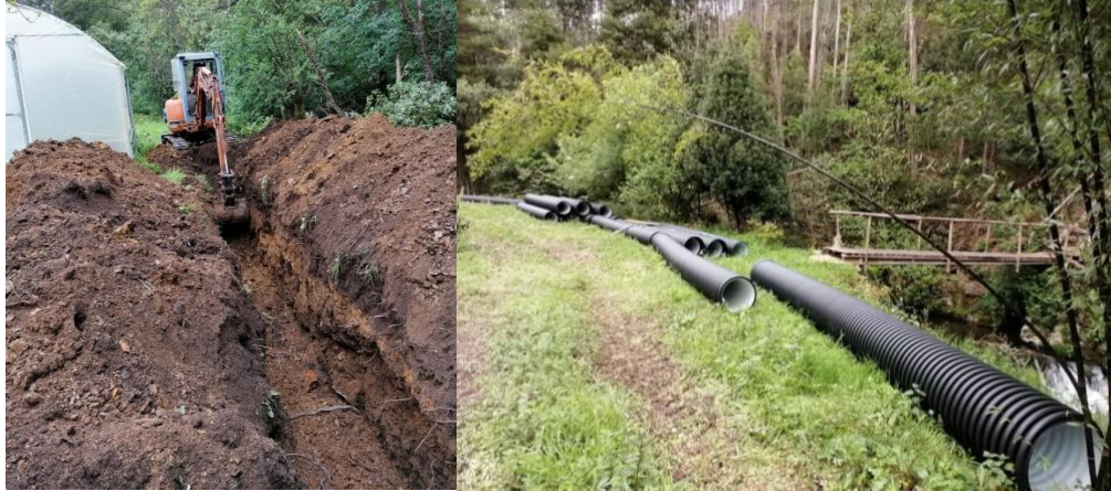
Figure 18. Pilot plant in the agro-tourism centre in Portugal.
