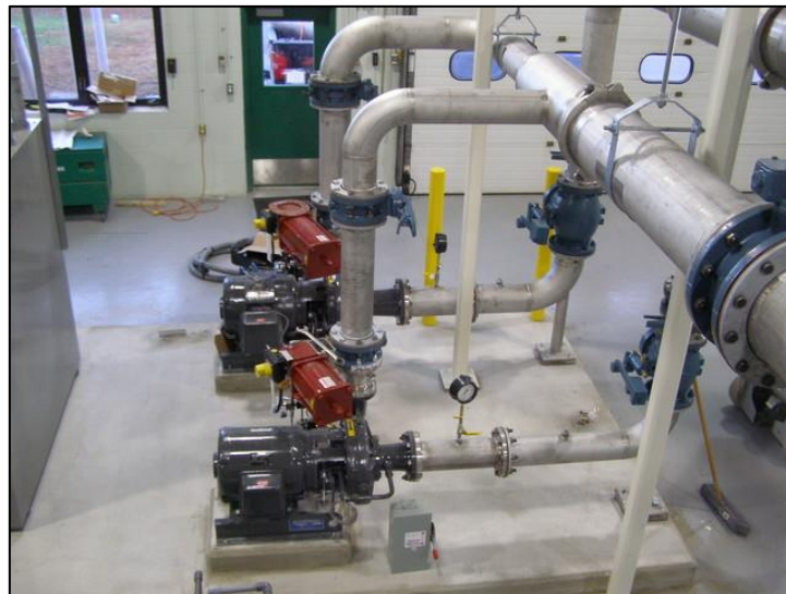
Turbine installation in UK water treatment works
