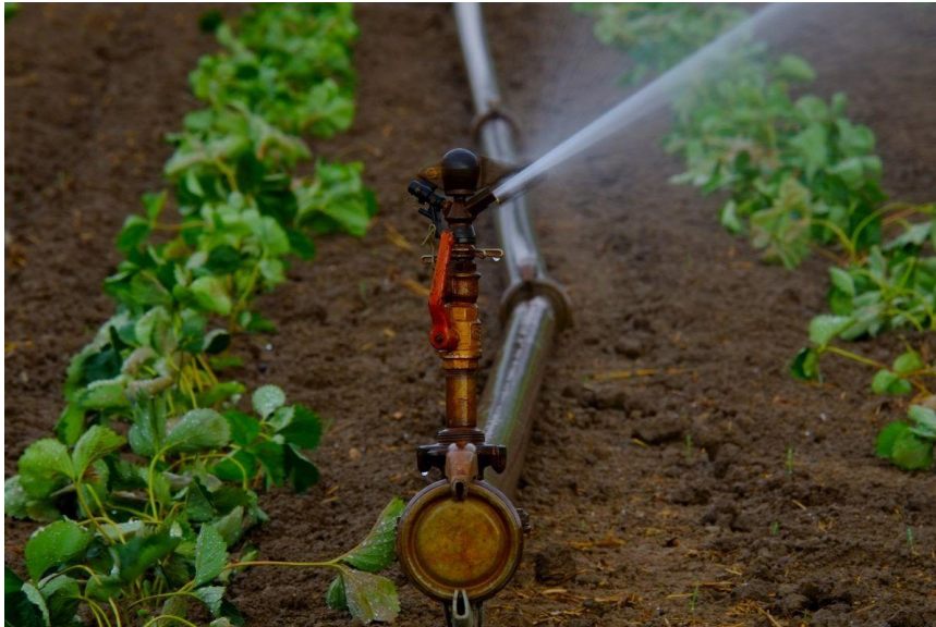
Detail of an irrigation system
