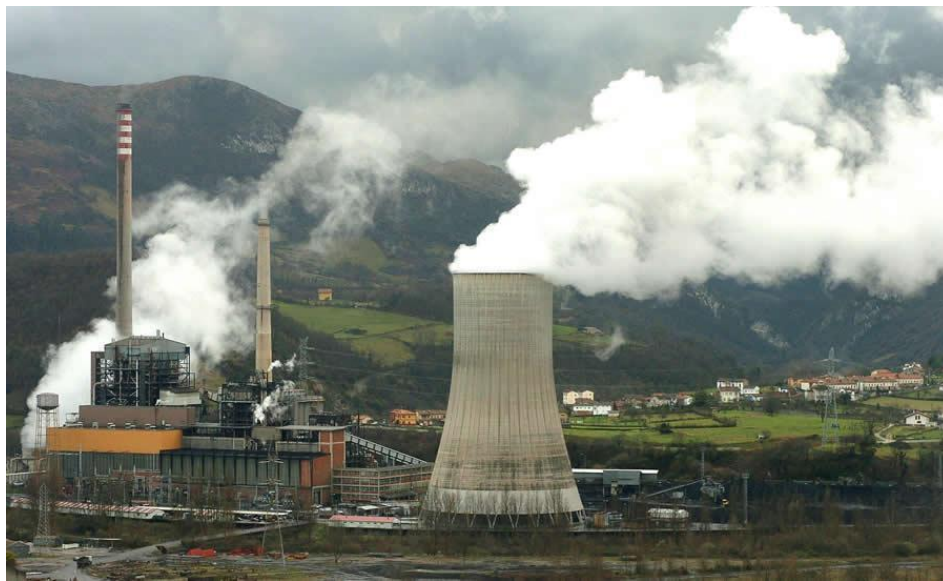
A thermal power plant
