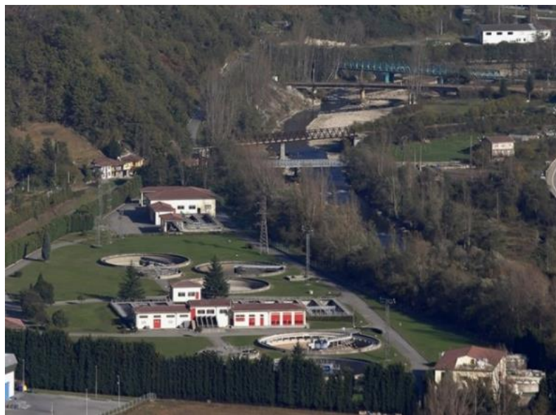
Wastewater treatment plant in Spain
