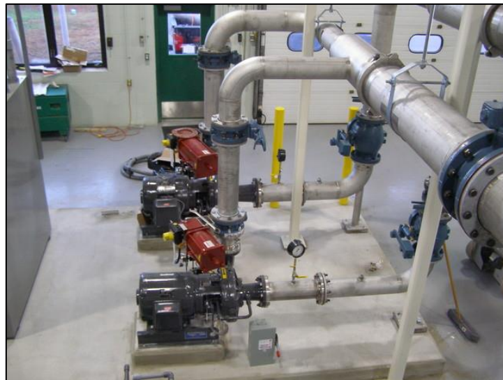
Turbine installation in UK water treatment works
